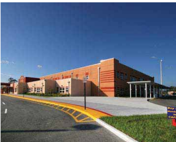
Drop off area along curb- school would like additional covered area
